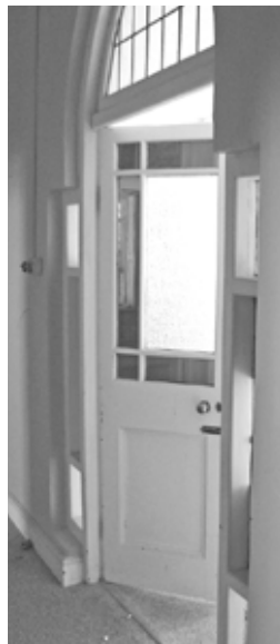
Above: A lost feature of the internal structure.
